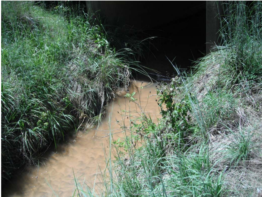
At station RYC-3 on Rocky Creek, looking upstream
