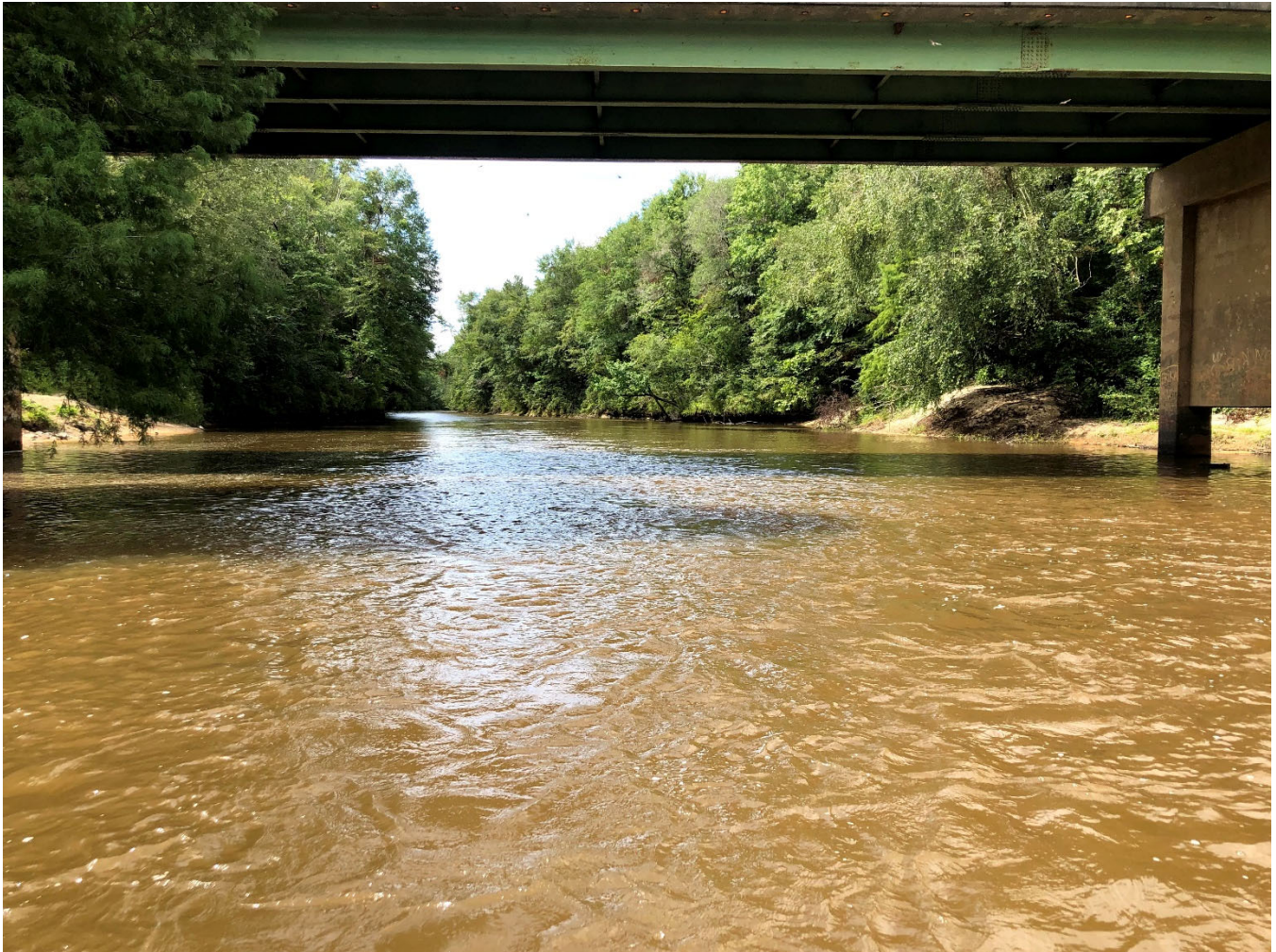
Station PEAC-3, Looking Downstream (7/8/2020)
