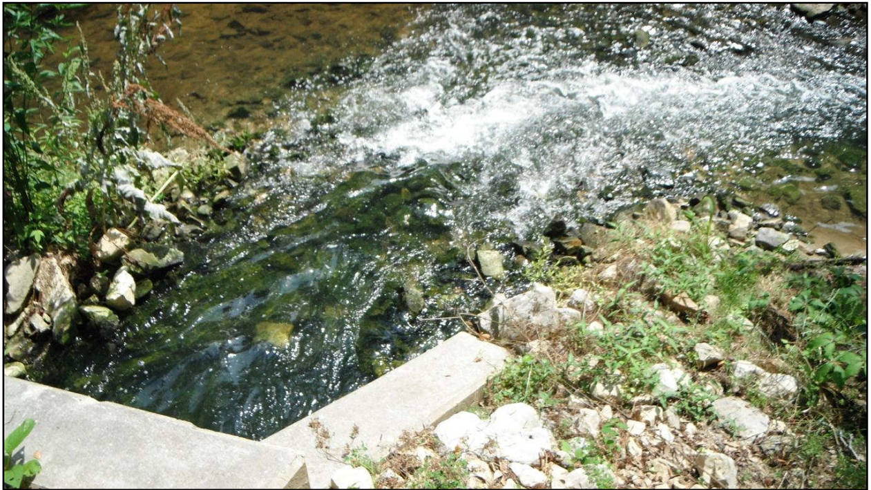
Picture 7: H.C. Morgan Outfall
