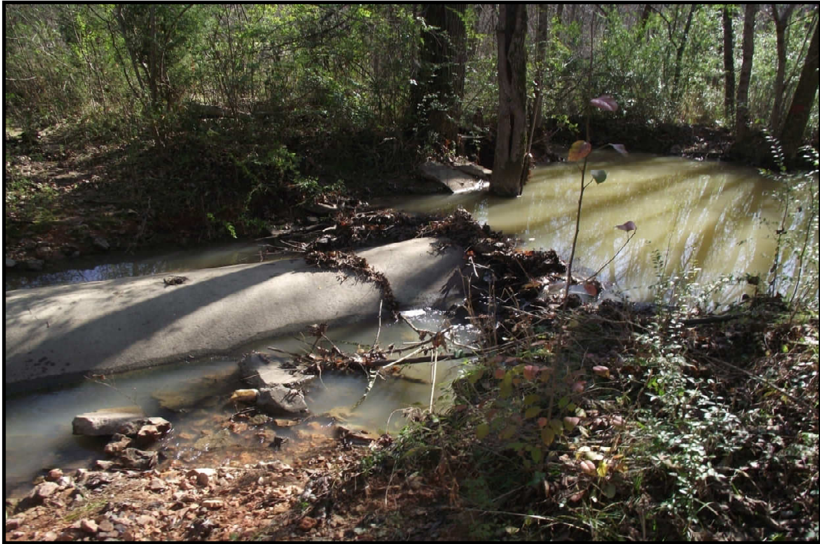
Culvert at LEBS-1. CPR & Steve Bearss. 12/3/10.
