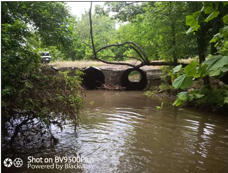
Figure 7.4.2: At Station PYCF-1: Downstream View (6/12/2023)
