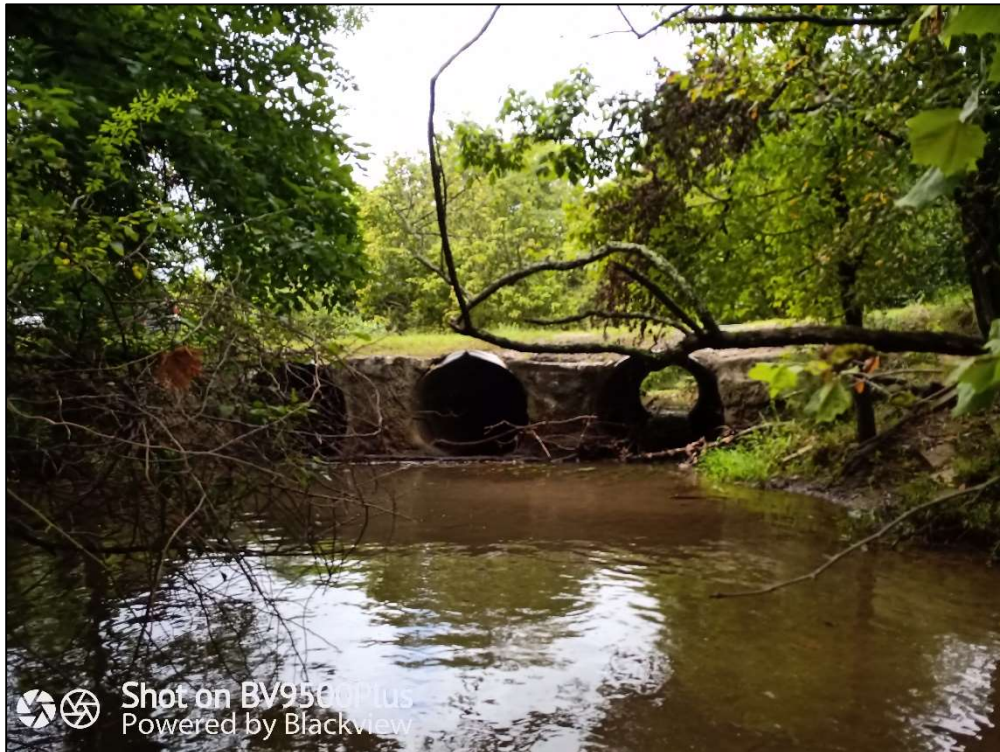
Figure 7.4.6: At Station PYCF-1: Downstream View (8/28/23)
