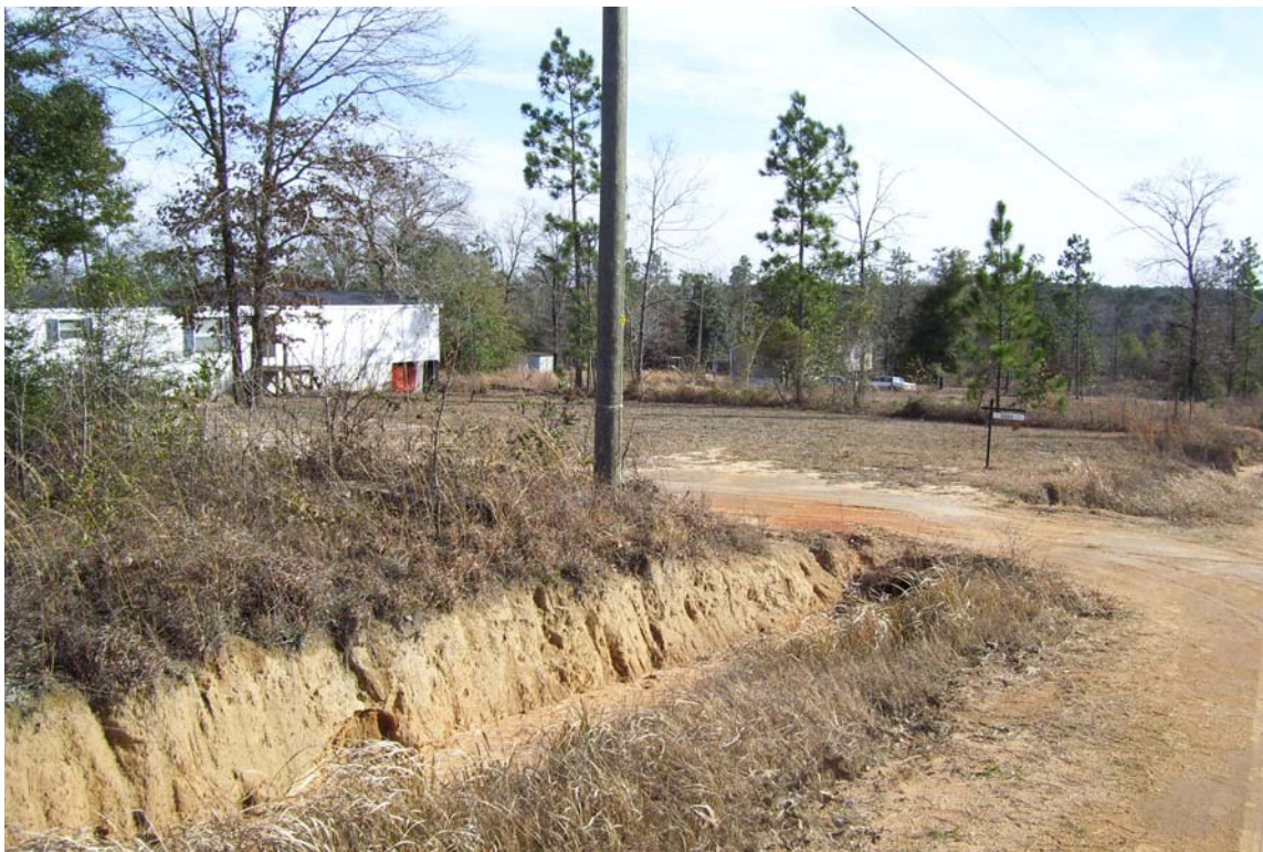
Photo 7-6: Mobile Homes and Drainage Ditch on North Bank of Collins Creek
