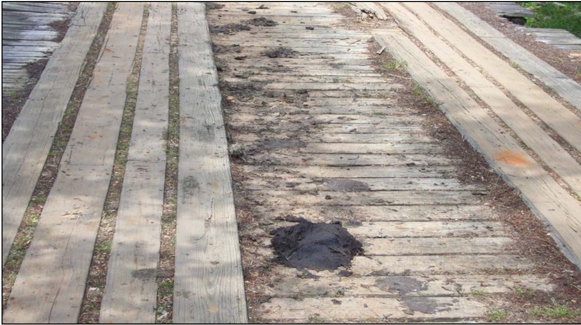
Figure 7-9: Fecal Matter on Bridge Crossing Bassett Creek at the Same Pastureland
