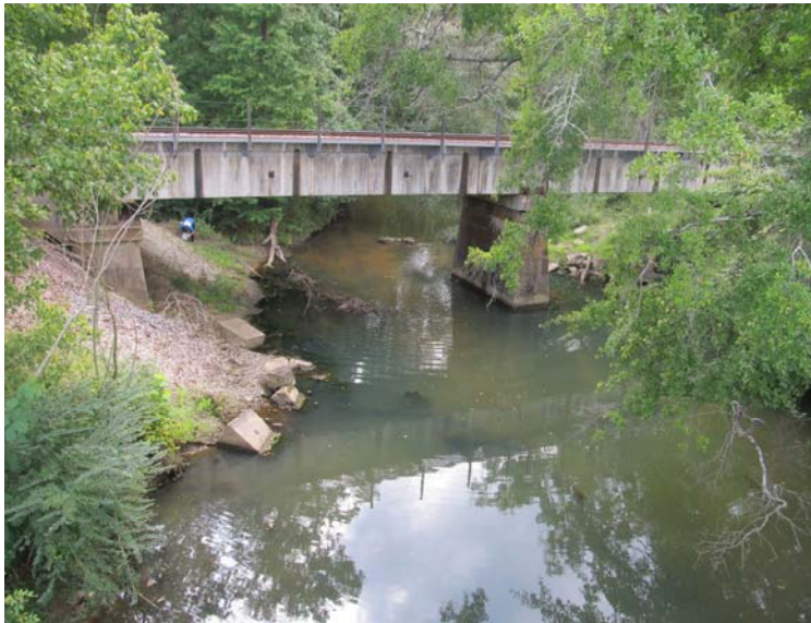
Figure 1. Lost Creek at LOSW-5, September 12, 2012.
