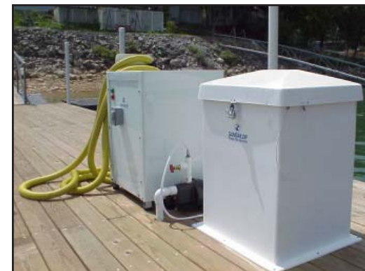
Pumpout and dump station combination.
