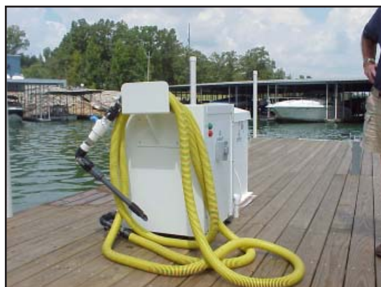
Pumpout station with wand attachment for portable toilets.
