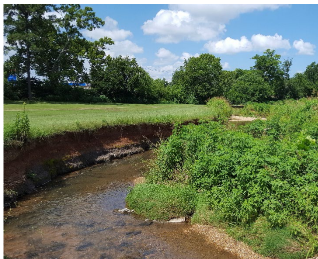
Figure 32. Village Creek at Roebuck Municipal Golf Course, identified as a critical area for bank stabilization
