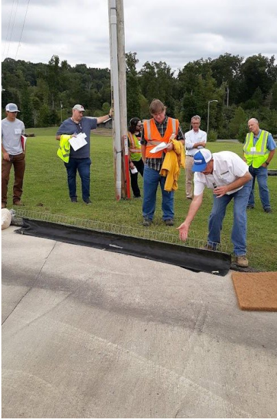
Figure 22. BMP installation demonstration
