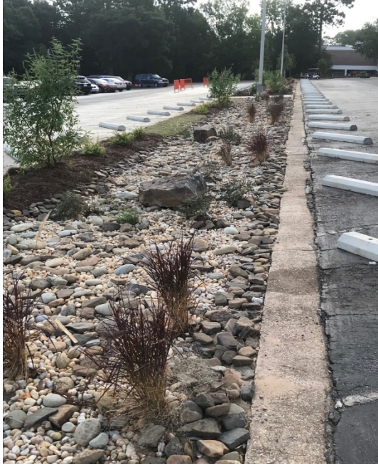
Figure 40. Bioinfiltration swale in the USA Humanities parking lot
