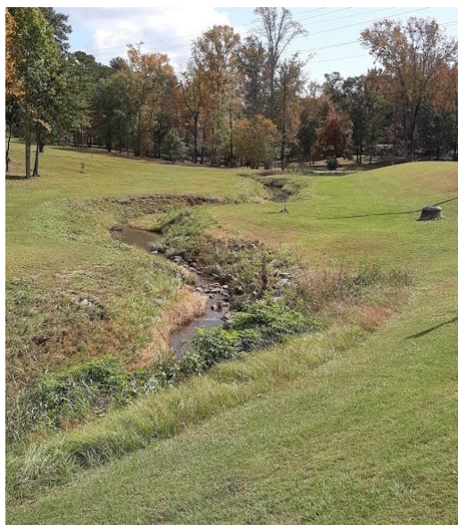
Figure 48. UT to Shoal at Sparkman Park adjacent to the baseball fields
