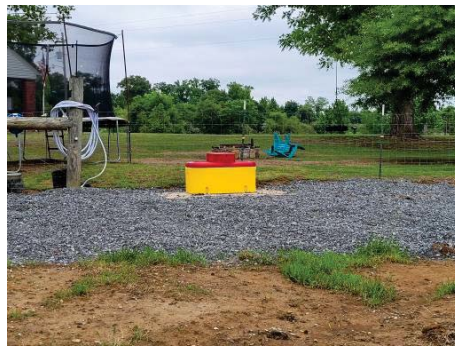
Figure 31. An alternative water source installed as part of the Graves Creek Phase II project
