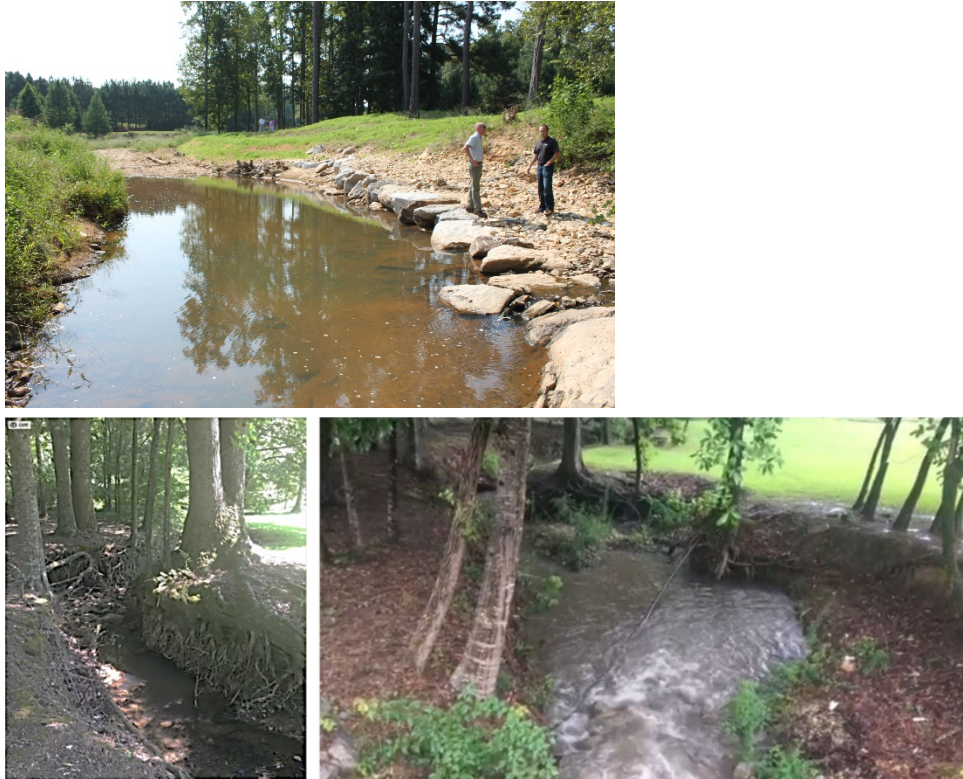
Figure 27. Golf Course BMPs implemented in 2008 (top) and headwaters in Hamilton Gables show evidence of flashy nature and streambank erosion (below)
