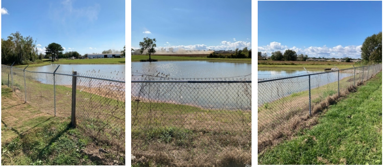
Figure 43. Stormwater detention retrofit at the City of Daphne Public Works Facility
