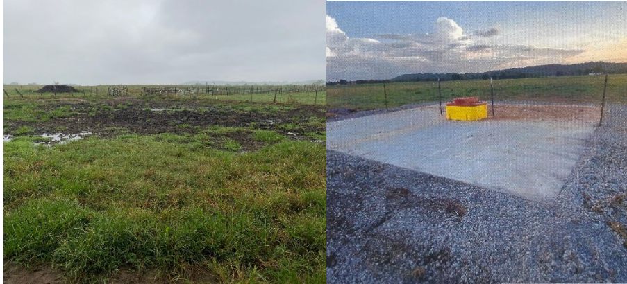
Figure 46. Alternative water source and heavy use area before (right) and after (left) installation
