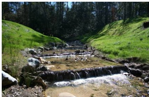
Figure 26. Restoration in D'Olive Creek constructed by Volkert, Inc.
