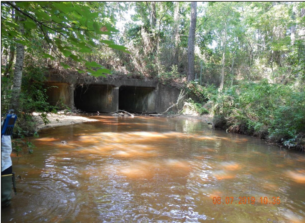
Figure C.4 Joes Branch Station JOBB-2 Downstream (8/07/2019 10:35)
