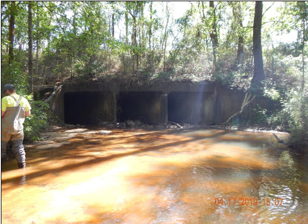
Figure C.2 Joes Branch Station JOBB-2 Downstream (4/17/2019 15:07)
