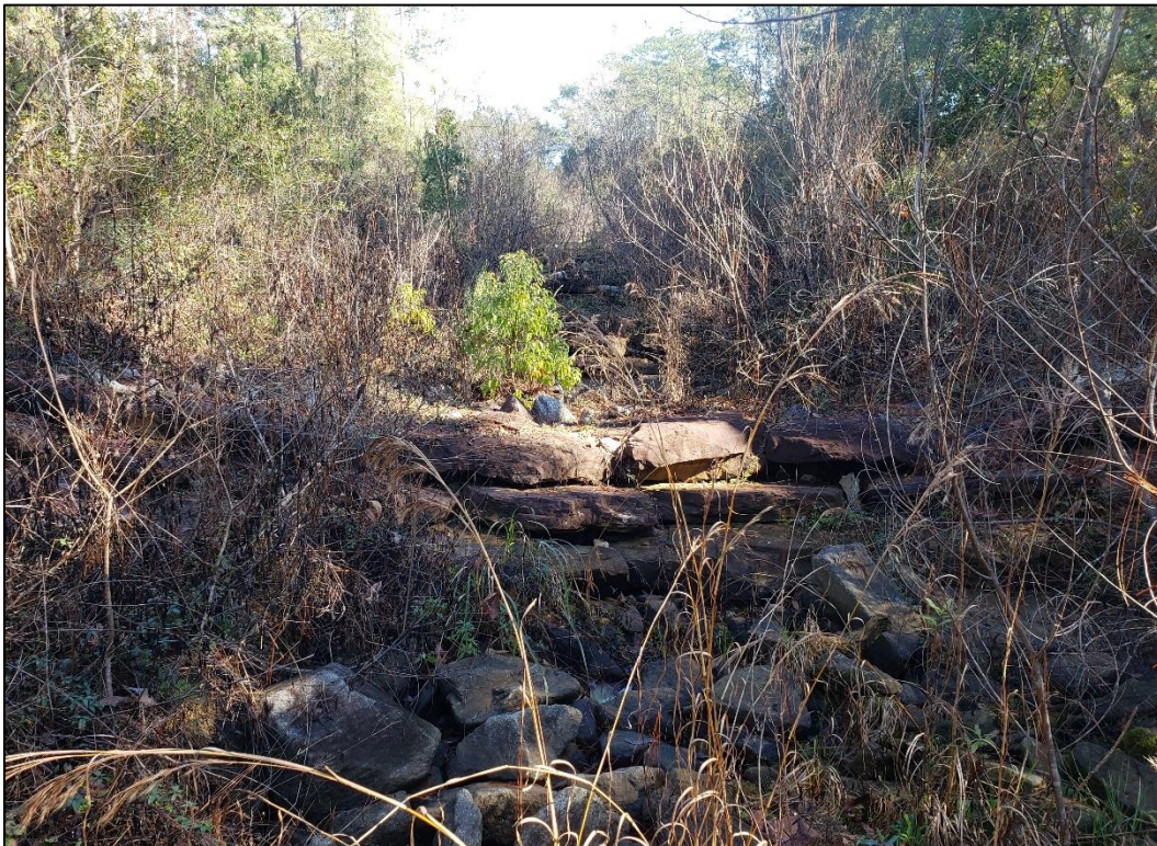
Figure C.10 Joes Branch UT 2012 Westminster Village Stream Restoration (Upstream)
