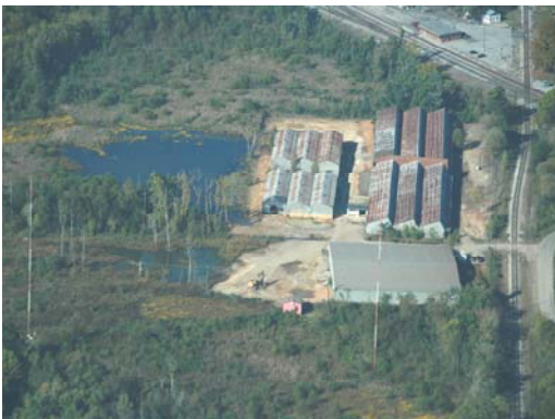
Four Star Wholesale Site (Etowah County) Post-Removal
