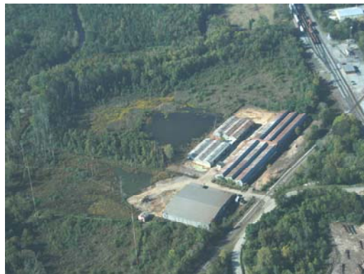
Four Star Wholesale Site (Etowah County) Post-Removal
