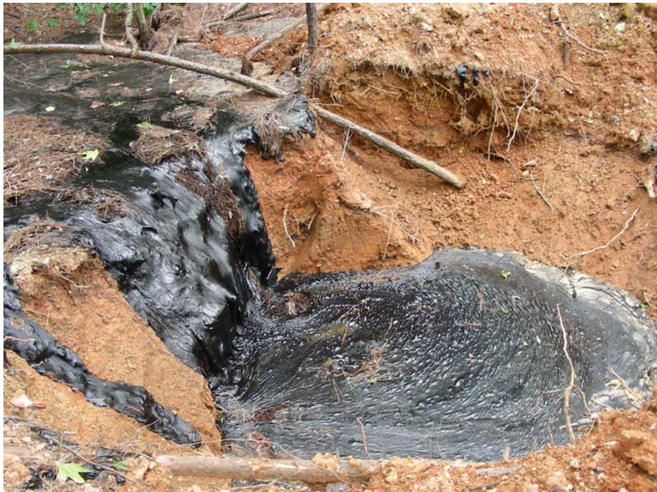
Lagoon runoff collection pit
