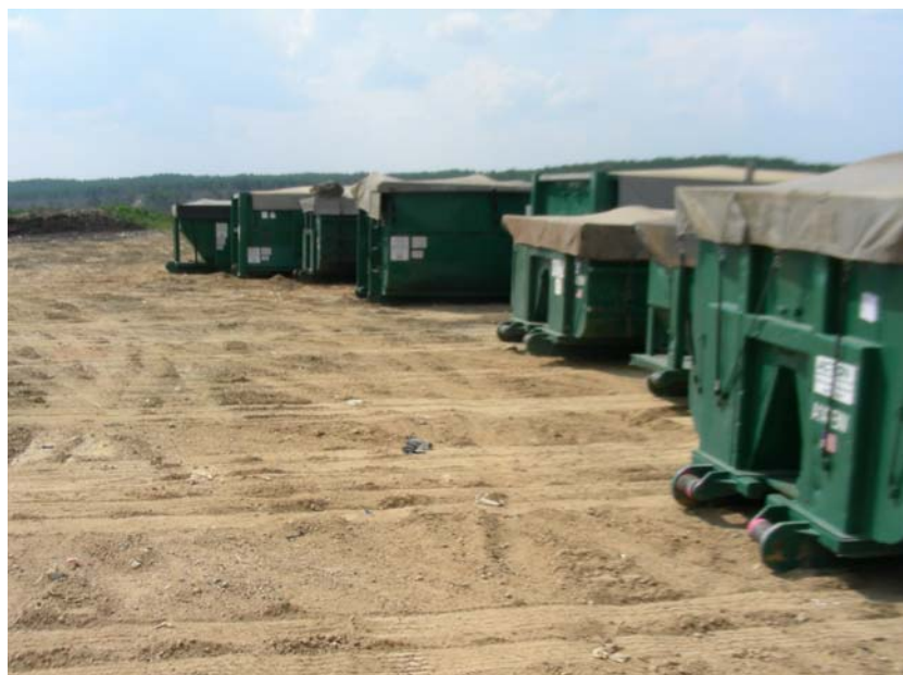
Roll-offs containing hazardous soil, staged for transport to Emelle
