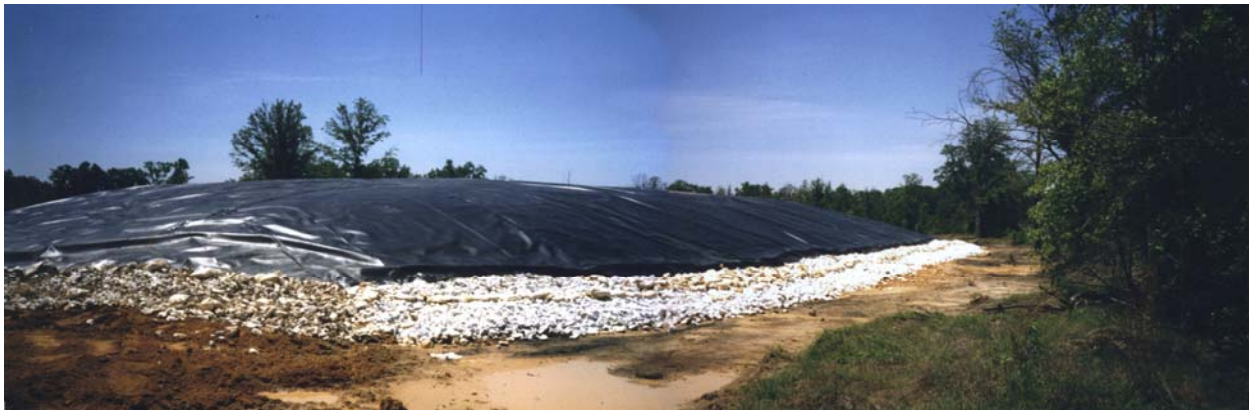
Brass foundry waste staged for removal
