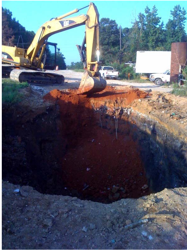
Excavation of the right-of-way along Highway 25
