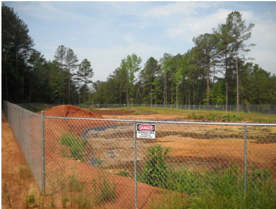
Completed slurry containment wall and enclosure
