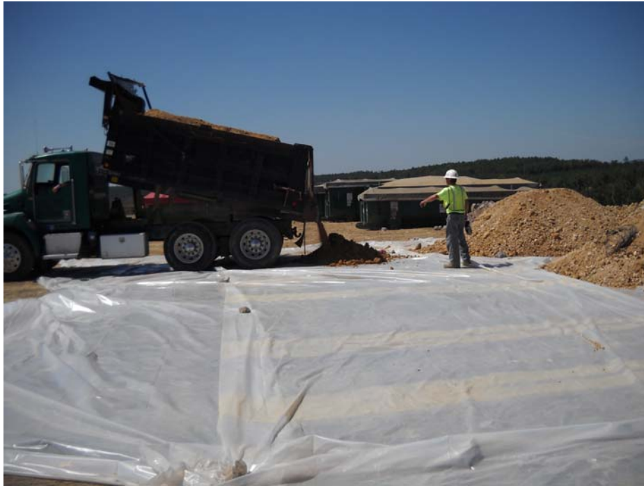
Non-hazardous surface soil removed from right-of-way
