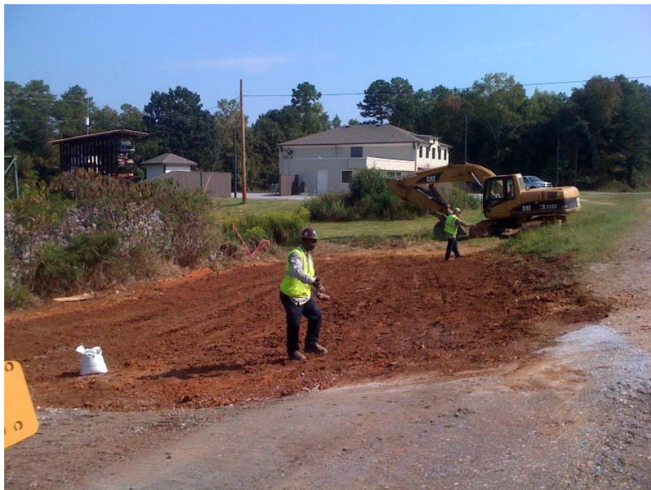
Backfilled excavation area with crew spreading grass seed
