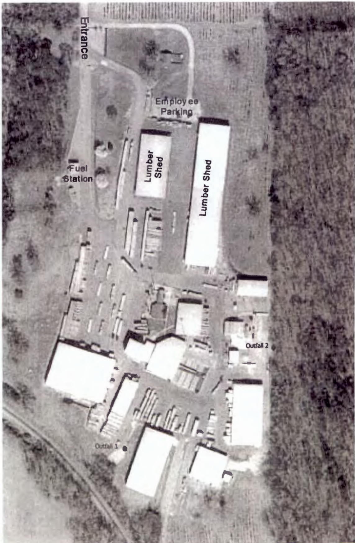
Southeast Wood Treating - Nauvoo, Alabama Stormwater Outfall Location
