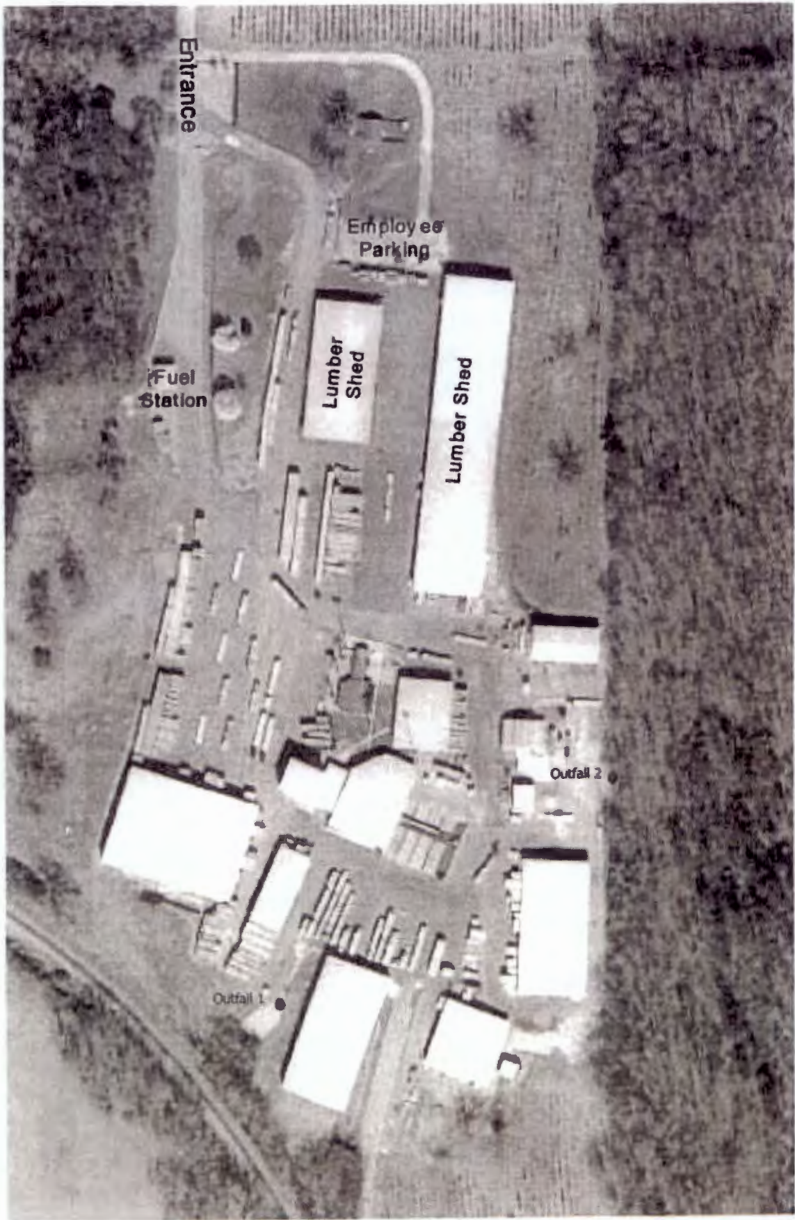
Southeast Wood Treating - Nauvoo, Alabama Stormwater Outfall Location
