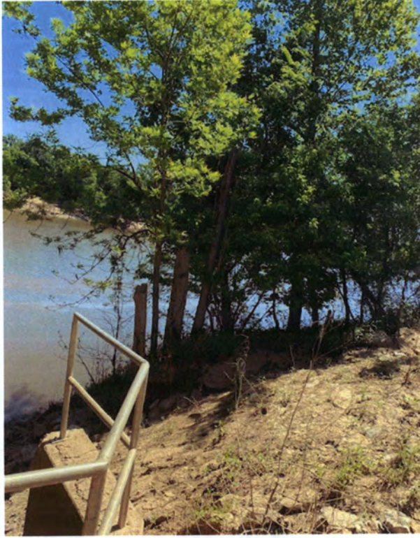
Figure 4. IP-Pine Hill Outfall, looking downstream
