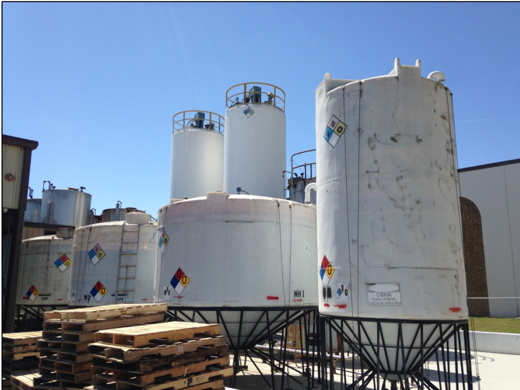
Tank System 1—Southwest View
