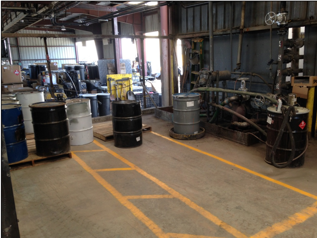
Waste Processing Area–Northwest View
