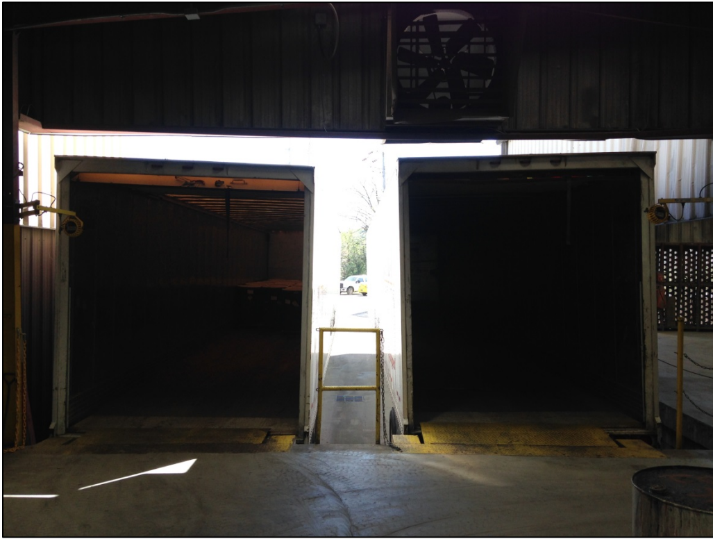
Container Loading/Unloading Dock–East View
