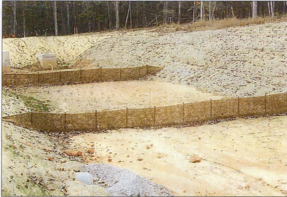
Figure SBN-2 Example of porous baffle made of 700 g/m 2 coir erosion blanket as viewed from the inlet. (from North Carolina Erosion and Sediment Control Planning and Design Manual.)
