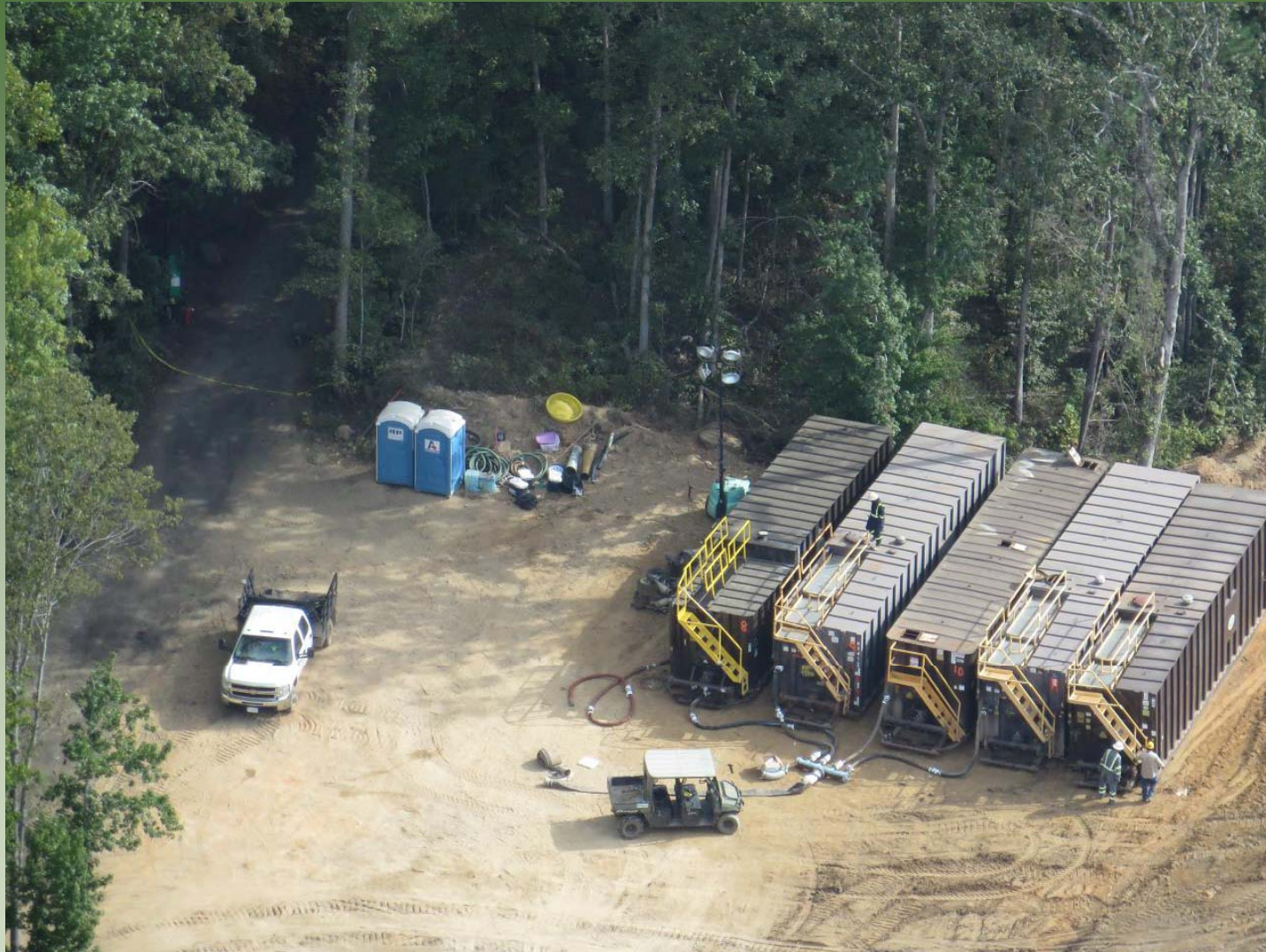
On-Site Frac Tanks Holding Petroleum Contact Water
