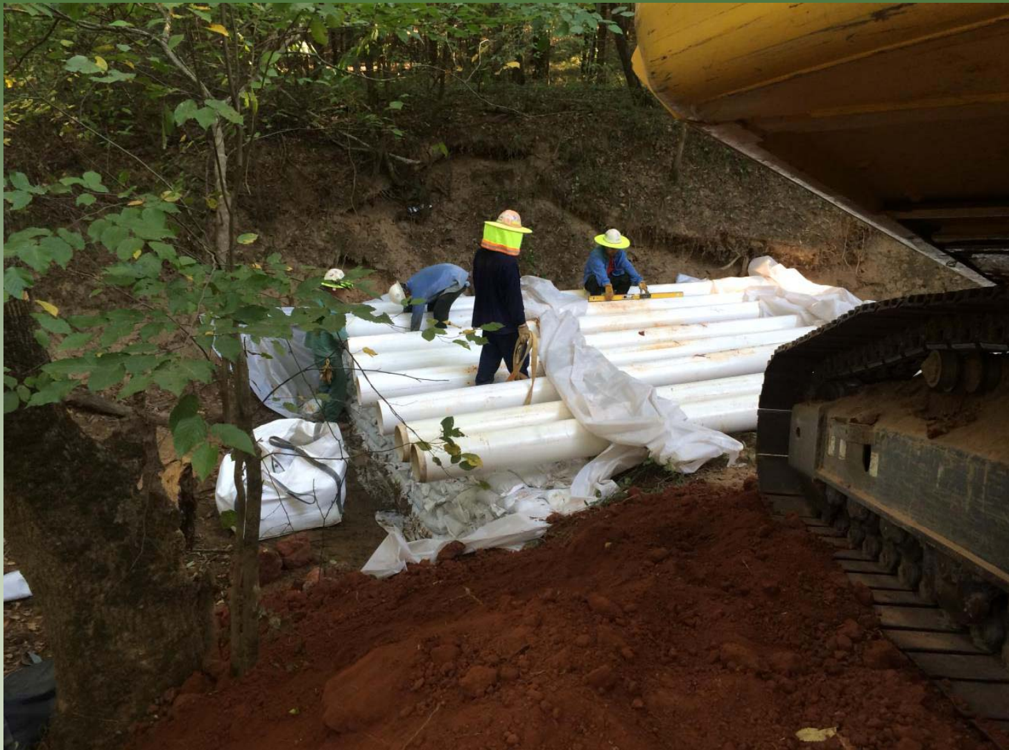
Underflow dam construction on Peel Creek using 18" diameter pipes
