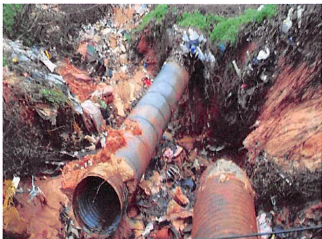
Lord Road, Dozier, Crenshaw County
