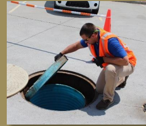
Inspecting a containment sump
