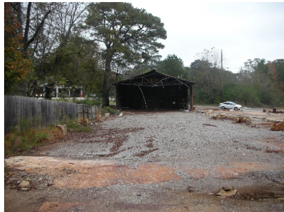
View to Shed from Back Fence
