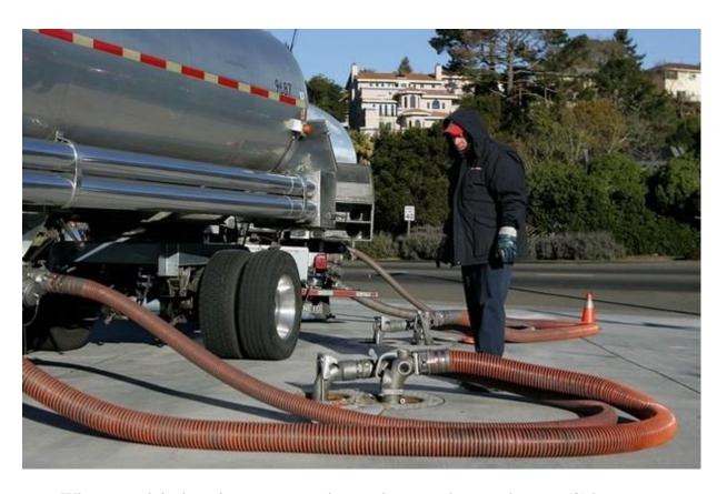
When a truck is dropping gas, remember to always make sure that two (2) hoses are used. One hose should be attached to the fill port, and the other should be attached to the vapor port. If you see ANY fumes or smell excessive gas odors, then inspect the adaptors for proper "hook up" and check the hose wall for tears and cracks. Also, please remember to look up at the pressure relief valves if possible to check for visible vapors.
