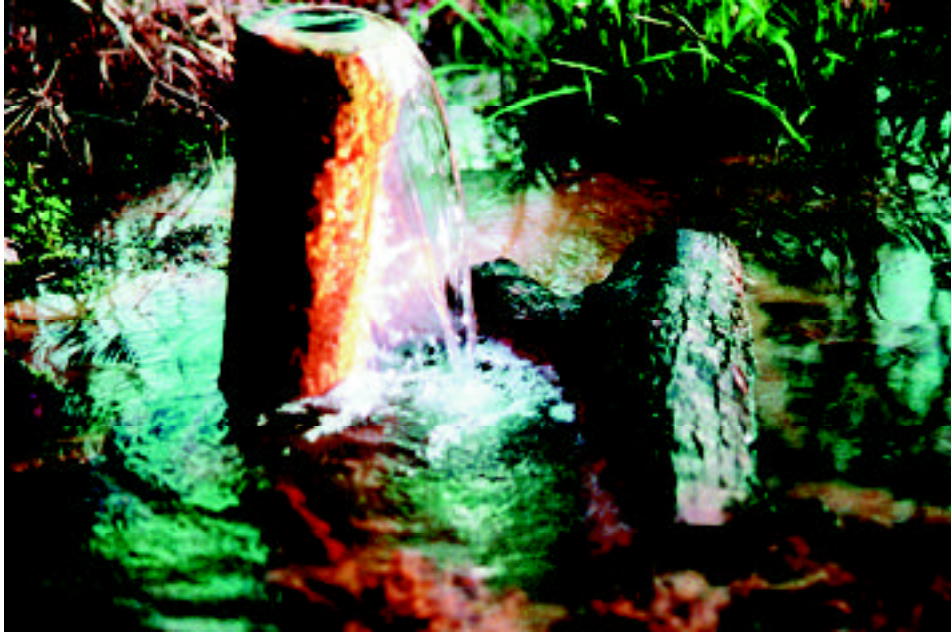
Flowing wells can waste millions of gallons of water. The rust colored material on the pipe is due to the iron content of the water.
