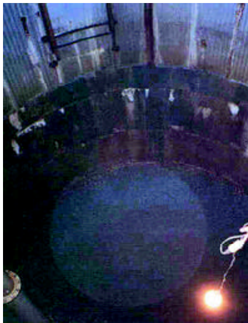
The Huntsville Lincoln Well is the largest diameter well (20 feet) in Alabama. It can pump up to 3200 gallons per minute.
